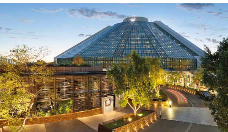
CROWN METROPOL PERTH
